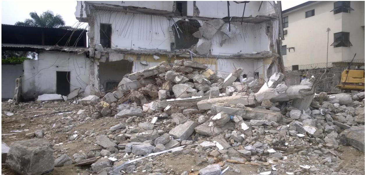
Figure 1: Building rubbles along Trans-Amadi, Port Harcourt, Nigeria.
